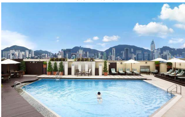
Rooftop outdoor heated swimming pool
